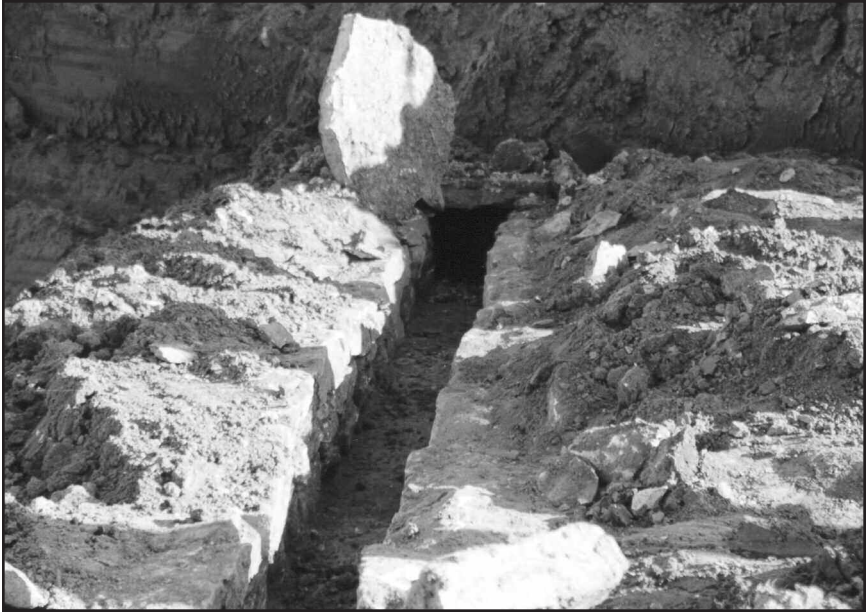
Figure 11. This additional portion of the Font Drain was located in 2000 when the foundations for the restored Nauvoo Temple were being dug. Courtesy NRI, photographer unknown.
