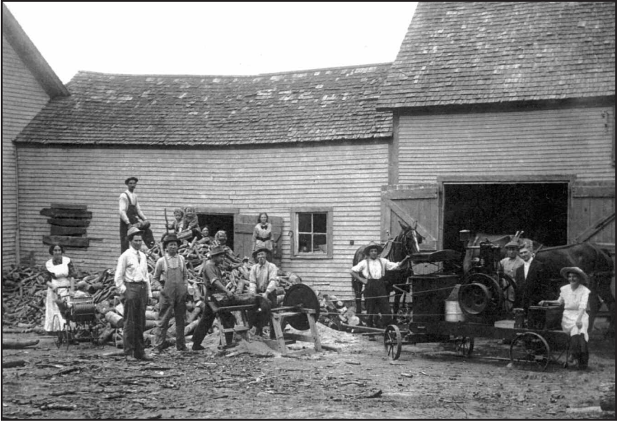
In the 1910s, the addition of agricultural functions transformed the site into the Joseph Smith Memorial Farm. Frank Brown stands in the left foreground with a necktie and hat, his wife, Winnifred, is seated at the far right.
